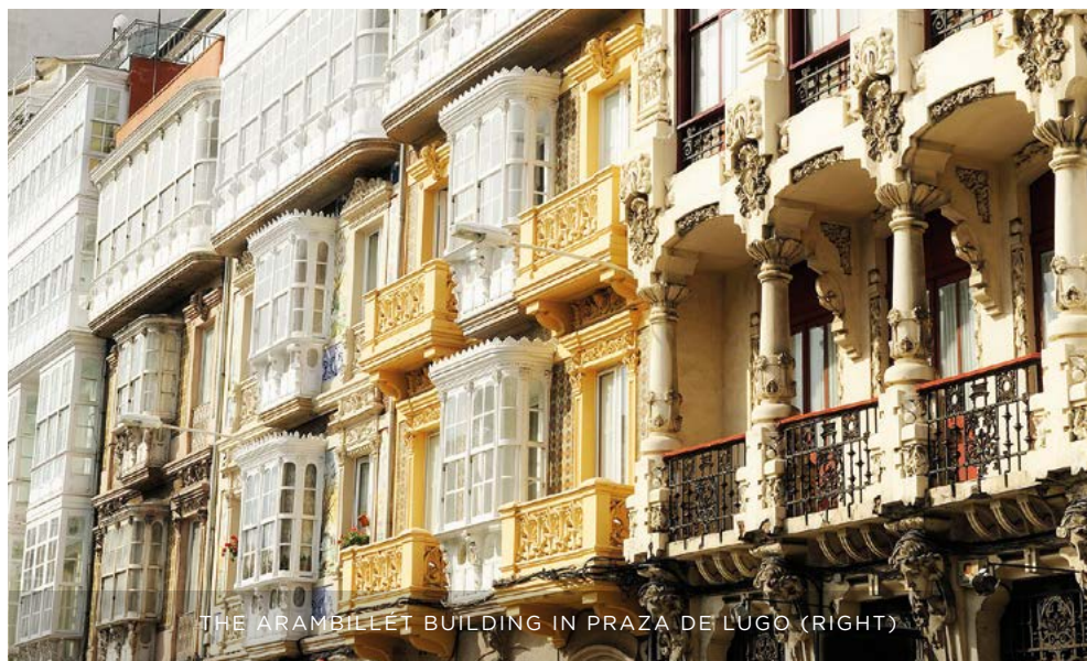
DETAIL OF A FAÇADE IN PRAZA DE LUGO
